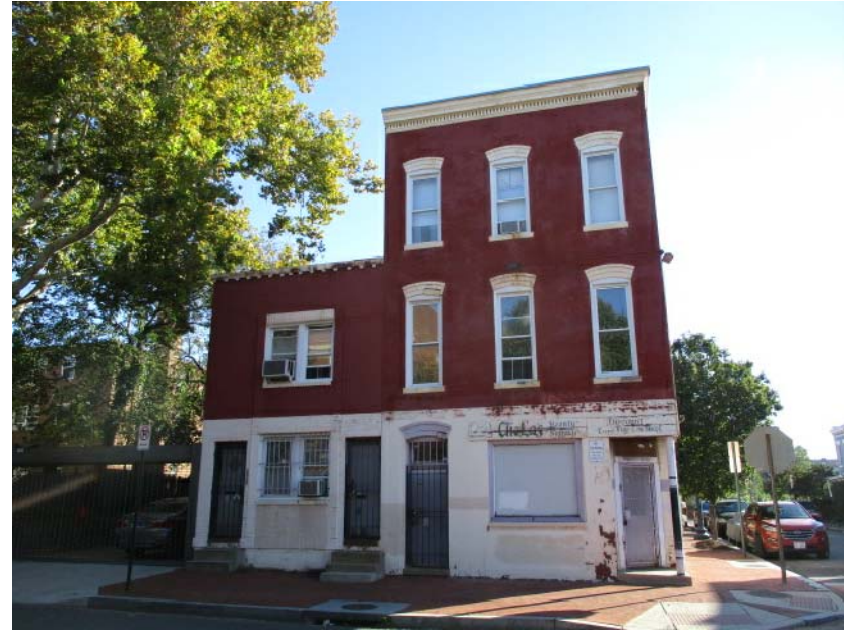
2. 2021 4TH STREET, VIEW EAST
