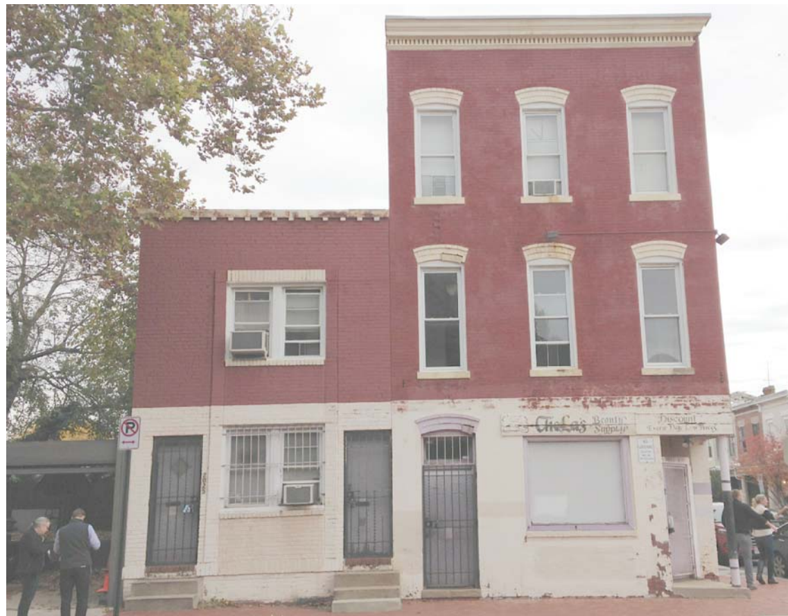
VIEW AT FRONT FACADE
