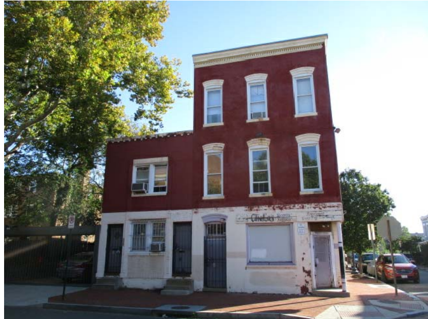
1. 2021 4TH STREET, VIEW EAST
