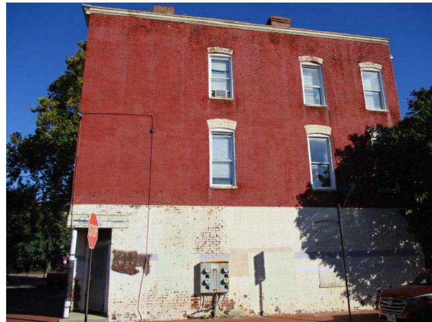
4. 2021 4TH STREET, VIEW NORTH
