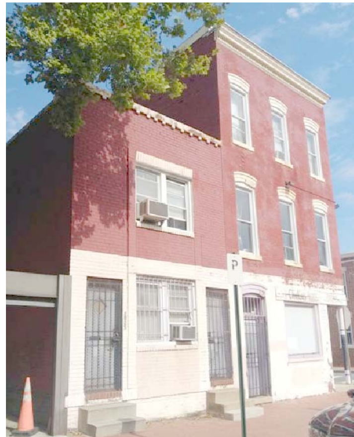
OBLIQUE VIEW AT FRONT FACADE
