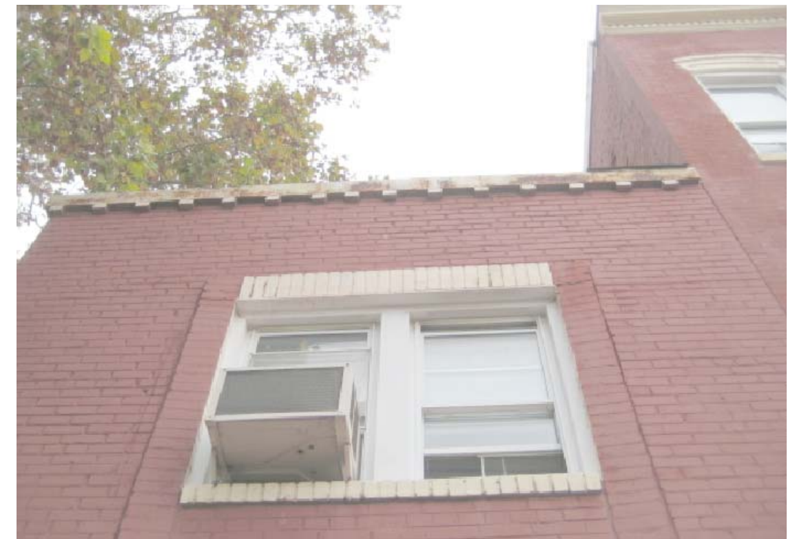
ROOF COPING - EXISTING CONDITION
